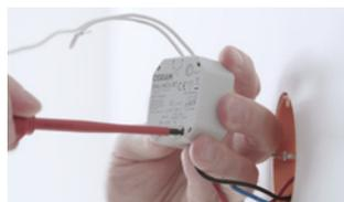
**01** Connect the DALI ACU BT to the mains wires as well as to the DALI wires of the LED drivers/ECGs.
